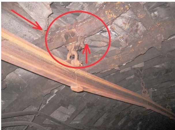
Fig. 1. Negative results of impact by dynamic loads of rolling SMR equipment of arching and the mine working roof [4]
