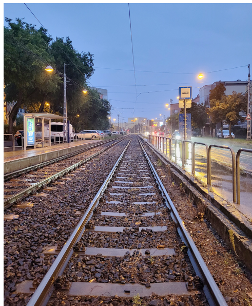
Fig. 1. The selected section – ballasted track (own photo)
