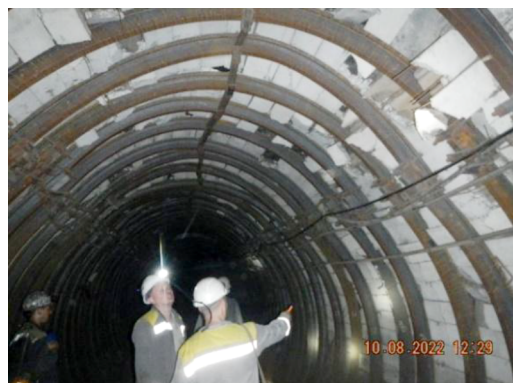
Fig. 2. Fragment of the state of the Western Main Ventilation Drift (PK 244)
