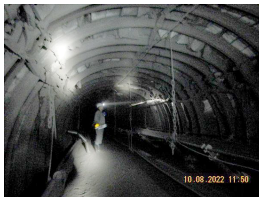
Fig. 3. Fragment of the state of the Western Main Conveyor Drift (PK 58)
