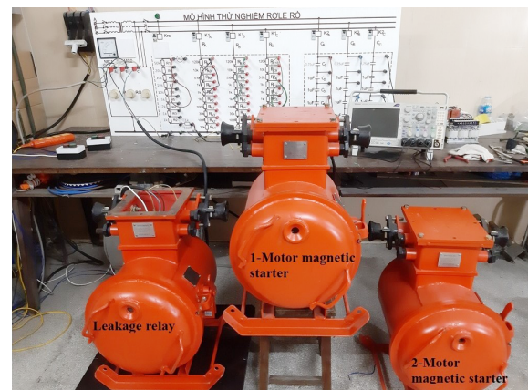
Fig. 2. Lab setup of devices for earthing resistance measurement with two motors which are wired to earth
