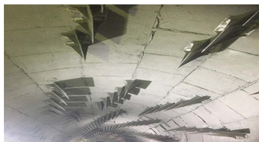
Fig. 9. View of shovels inside rotary kilns at Ferronikeli Plant in Drenas (June 2019)
