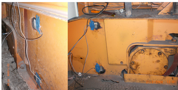
Fig. 5. Installation of strain gauges on the crane end beam
