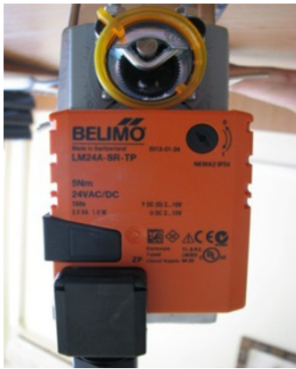
Fig. 2. Electric drive Belimo LM24A
